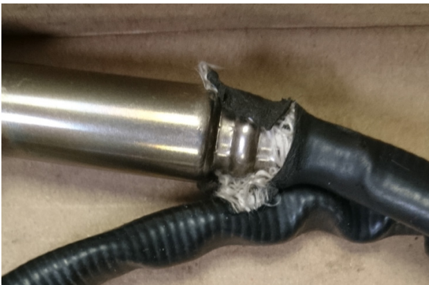
Figure 14. Evidence of damaged wiring.
